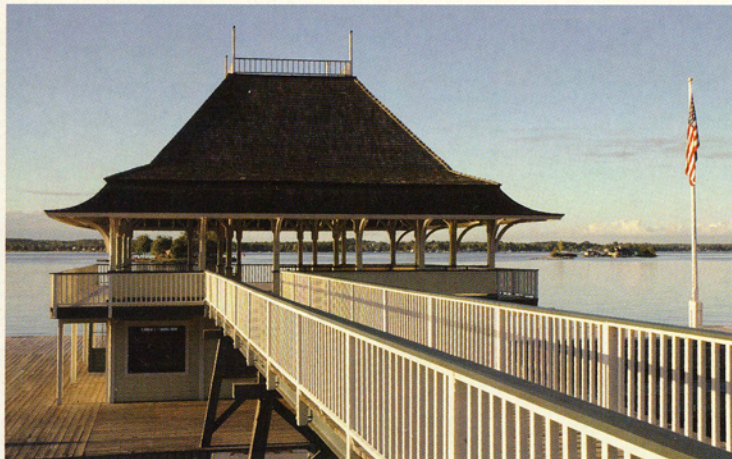
Resting in the morning sun is the Thousand Island Park Pavilion. This restoration project was designed by Steve Taylor in conjunction with Grater Architects.
